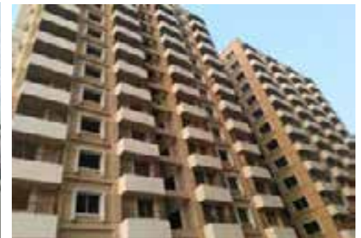
● Shopno-Nagar Housing, Dhaka (Photos: Chowdhury, Web source)
