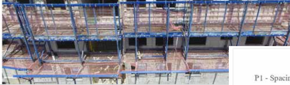
b) Temporary work platform with guardrails
