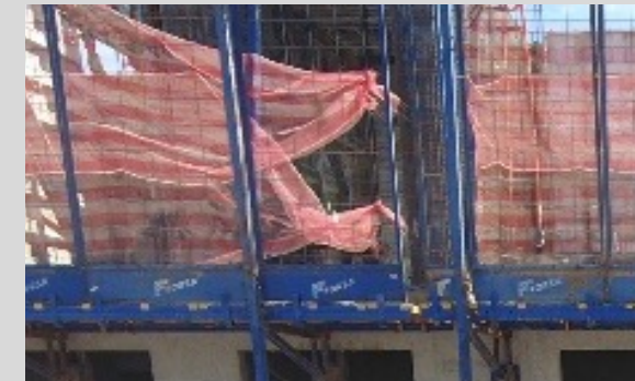
Openings in the screens fixed to the panel
