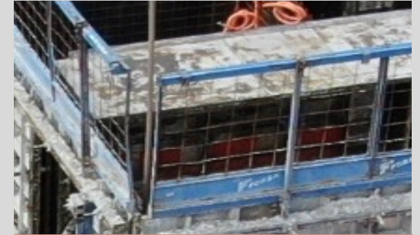
Spacing between guardrail elements
