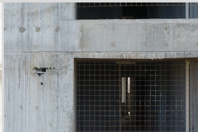
Exposed reinforcement
