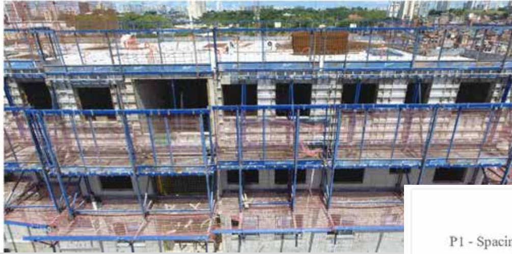
b) Temporary work platform with guardrails
